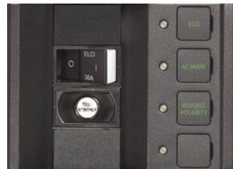
Residual Current Circuit Breaker (p.87)
