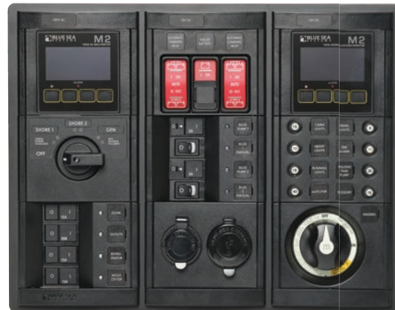
Completed 3 x 3 Panel
